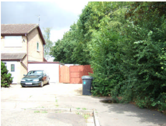
Fig 11: Trees encroaching towards a residential property.
